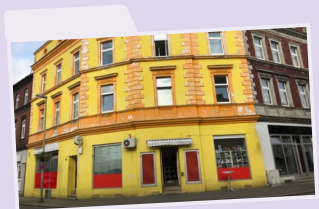
Problemimmobilie in Essen
